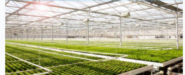
Construction of a greenhouse complex
