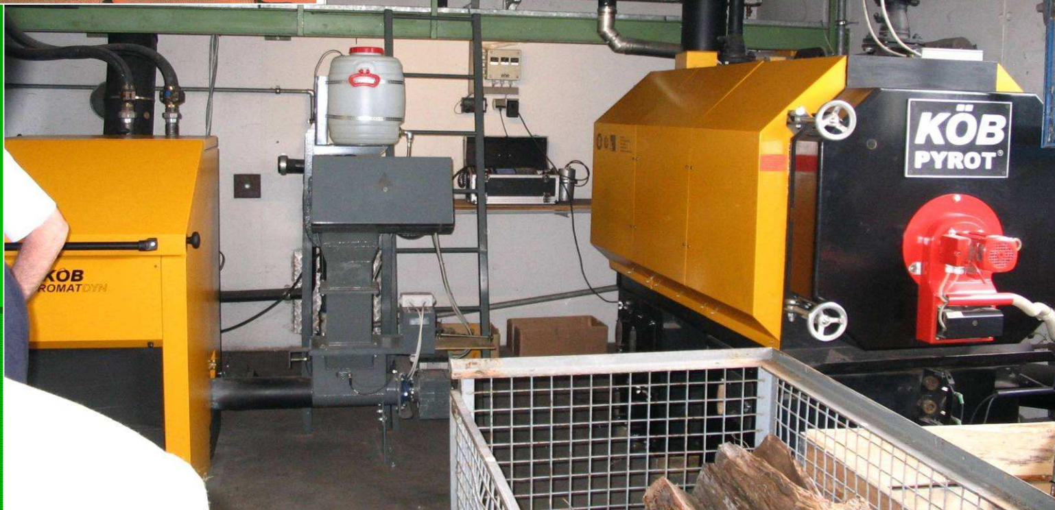
PYROT plant (250 kW) for ground timber firing
